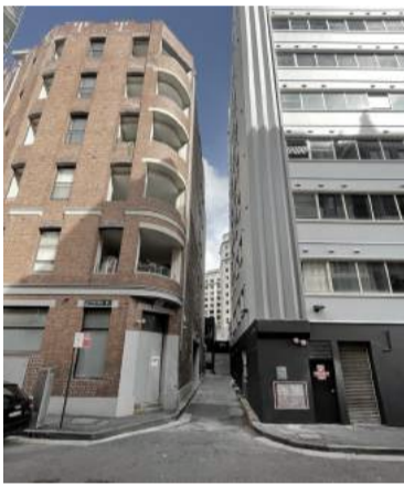
Foster Lane (Subject Site at end of lane)
